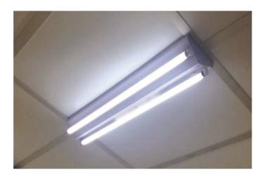
MYLED's BroadLumen Plus is easy to install and has up to 4 times the life span of a traditinal T8 fluorescent tubewith the added benefit of containing non harmful mercury content.
